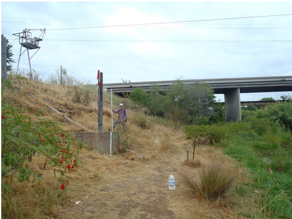
Figure 6. Bear River near Wheatland (RM 11.5, USGS gage 1142400). Stadia rod is being held at the 1.5 yr. recurrence interval at staff gage elevation of 6.45 ft. (2,656 cfs).
